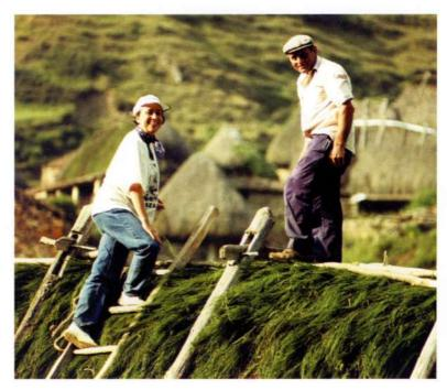
Advocates of the first method argue that the broom tends to rot under the long timbers, which prevents ventilation in the thatching. The first technique is preferred in areas located at a higher altitude, but it is obviously also a question of local idiosyncrasy in the communities of the different valleys.
