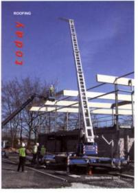
The Front Cover depicts a self operated TC28 trailer mounted crane positioning roof materials. This trailer crane is part of the largest fleet of trailer mounted cranes in the UK. The fleet is operated by Oktopus UK Ltd
